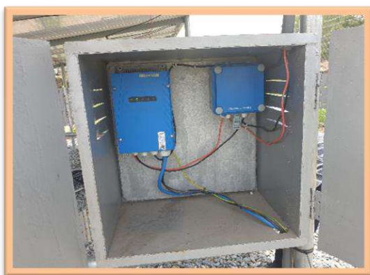
Photo 8: Control devices of a solar-powered irrigation system in protective box that can be locked
