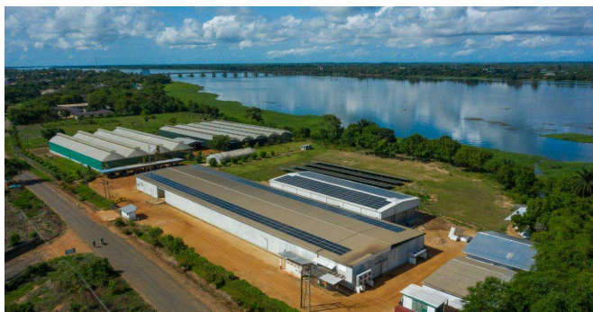
The recommended investment of approximately €500,000 has been secured by Iribov Ltd. The 400 kWp solar installation has been completed after 3 months of installation works in May 2023.
